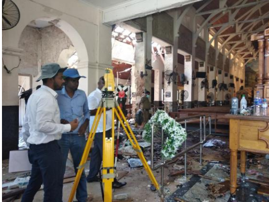
Figure -1 Survey for further Investigation, After the bomb blast At Kochchikade--2019
